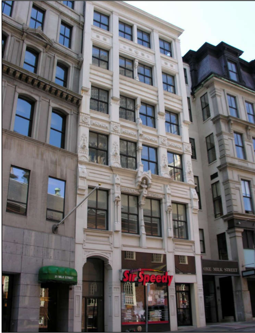
The site of birthplace is commemorated by a bust above the second floor facade of this building.
